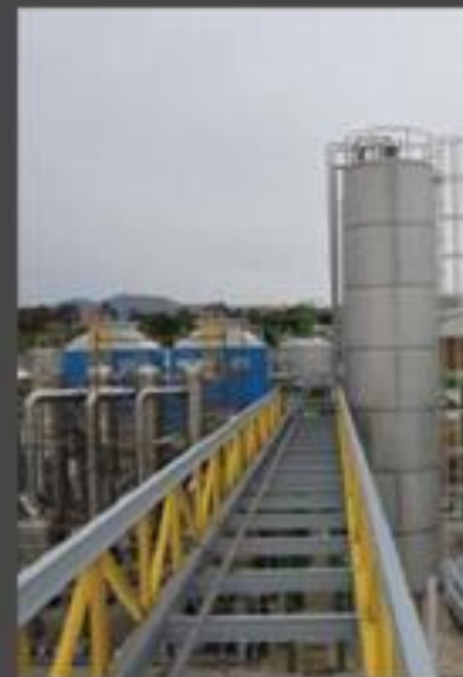
ALTACA Environmental Technologies and Energy Inc. / Turkey
